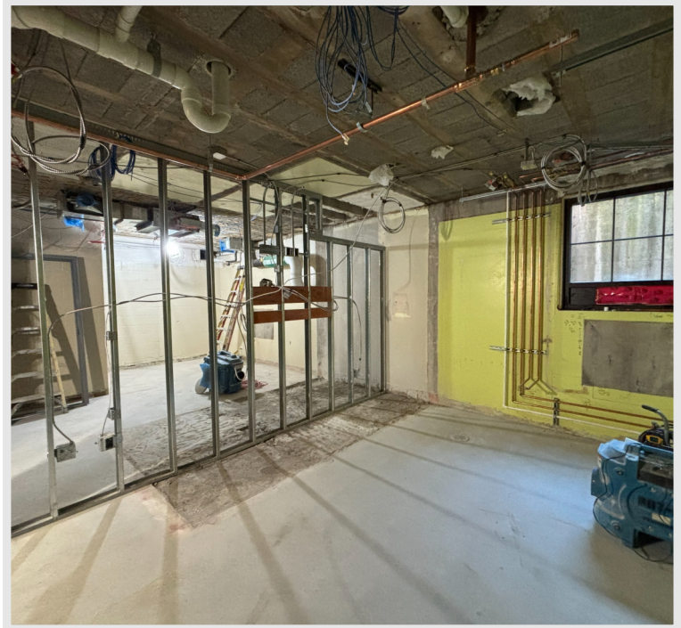
Masonry and stud wall framing is complete in the Lower-Level ELL/SGI Rooms, while MEPF overhead rough-ins continue above.
