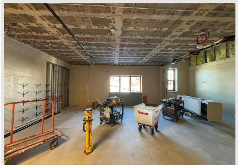
Overhead rough-ins nearly complete in the Second-Floor 3 rd Grade Classroom. This space is ready for drywall and finishes starting soon!
