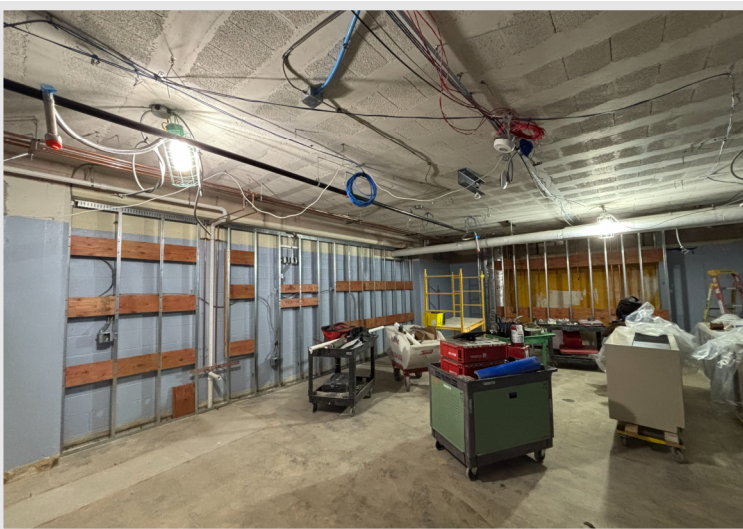
Wall framing, rough-ins, and blocking in place in the Lower-Level OT/PT Room. Overhead MEPF rough-ins are moving along!
